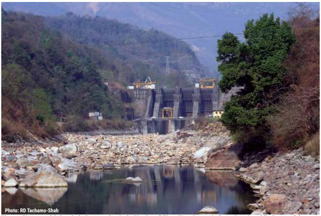
Photo 1: River stretch below the hydropower dam in the Marshyagdi River. Water is seen in the pool section while the rest of the dewatered zone is dry.
